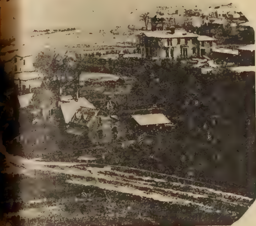
and the year 1870, Hall, an early home of the Varsity, which was later pulled down for the construction of the Biology building. Farm land surrounded the campus in those days.
